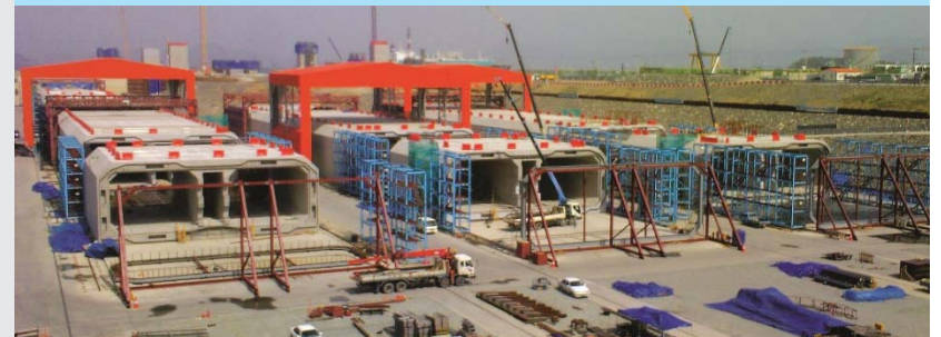
Geoga Grand Bridge (Republic of Korea)
