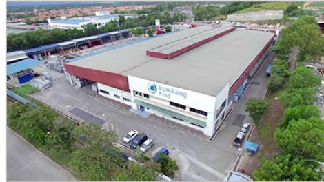
2009. 10 Completed Nilai Factory Malaysia
